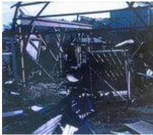
Photo of Deputy’s Cabin after Box Flat explosion
